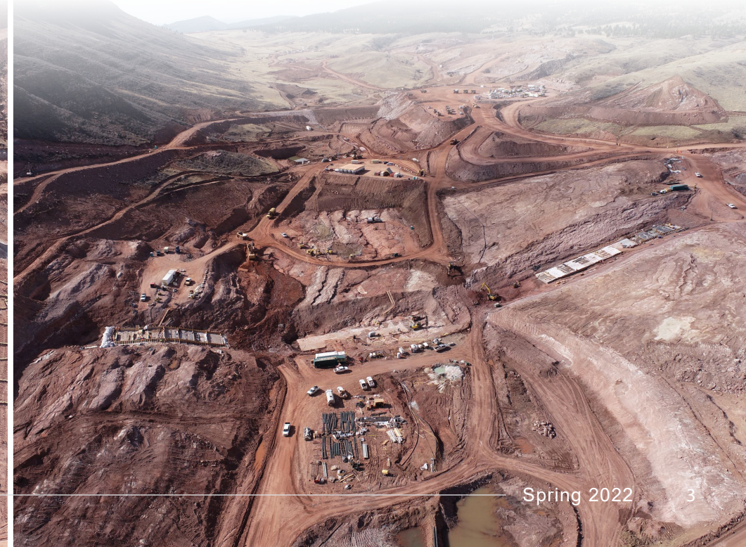
Right: The bottom 1,000 linear feet of core trench has now been exposed within the main dam, allowing plinth construction to commence.
