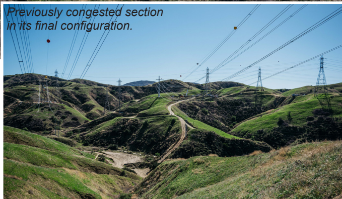
220kV corridor overlooking San Bernardino.
