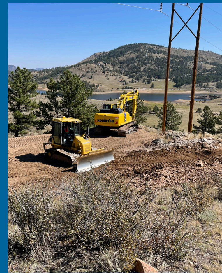
Top: Site preparation activities.
