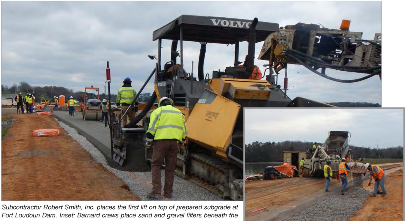
Subcontractor Robert Smith, Inc. places the first lift on top of prepared subgrade at Fort Loudoun Dam. Inset: Barnard crews place sand and gravel filters beneath the RCC subgrade using a material-placing conveyor.
