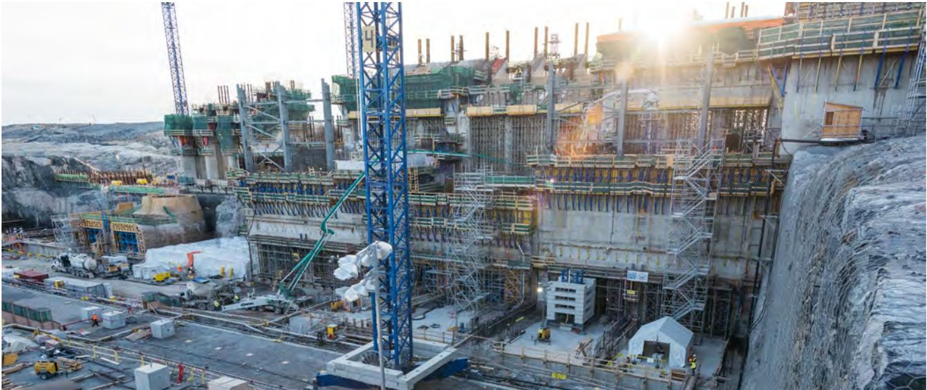
*A look inside the Keeyask powerhouse. Project construction includes a seven-unit powerhouse, seven-bay spillway, three zoned rockfill dams, two earthfill dykes, and cofferdams to reroute the river.*
