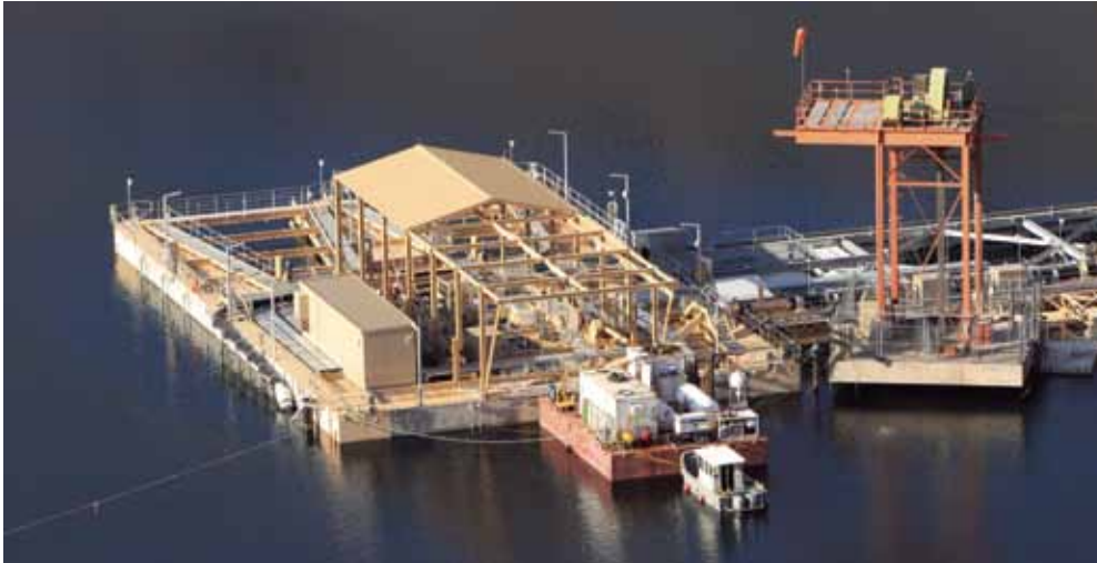
The recently completed Round Butte Dam fish screening and transfer facility sits atop a 270-foot-tall structure that helps redirect currents in central Oregon's Lake Billy Chinook.
